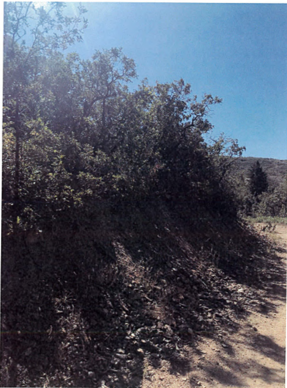
Photo 1: View along dirt road located in 30' Weber County ROW and 40' Utility Corridor looking south-east. Note erosion on east side of dirt road.
